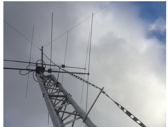
My balanced feeder system - wooden supports keep the ladder line away from the tower
