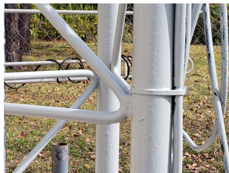
New paint job and new concrete base pad
