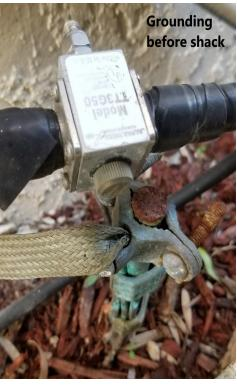
gear is grounded to that block using the flat braid wire. Where I didn't have a ground screw, as on my computer, I added one.
