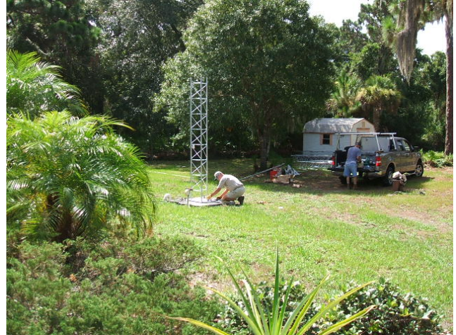
Julio Peralta – W4HY bolts down the first 10' section of Rohn 45G while Ron LeBrun – KB4RON gets the power winch ready to mount onto this section.
