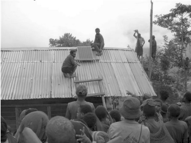
The solar panel is installed.
