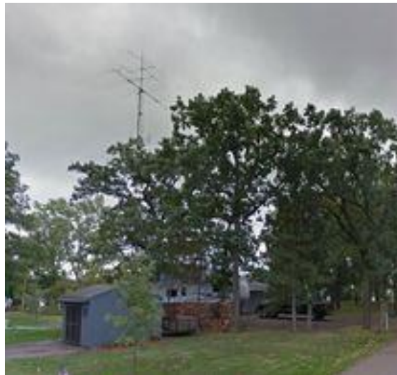
Tower involved in fatal fall
