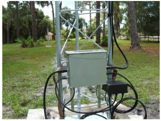
Interior view of lightning suppressors mounted on a Harger copper plate. The copper plate is bonded with two 1.5" copper straps to the adjacent tower legs and ground rods. The top suppressor is for the antenna rotator, with two coaxial cable suppressors immediately below. All suppressors are from Industrial Communications Engineers, Ltd. (I.C.E.).
