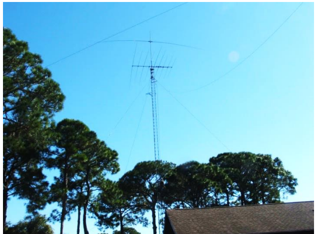
The Optibeam and 40m rotary dipole are ready to get busy working DX. The bracket at the 70' height is for a gamma match so that Al can load up the tower on 160m.
