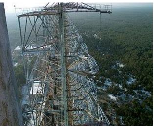
Duga-3 array outside Chernobyl. The array of pairs of cylindrical/conical cages on the right are the driven elements, fed at the facing points with a form of ladder line suspended from stand-off platforms at top right. A backplane reflector of small wires can just be seen left of center, most clearly at the bottom of the image.
