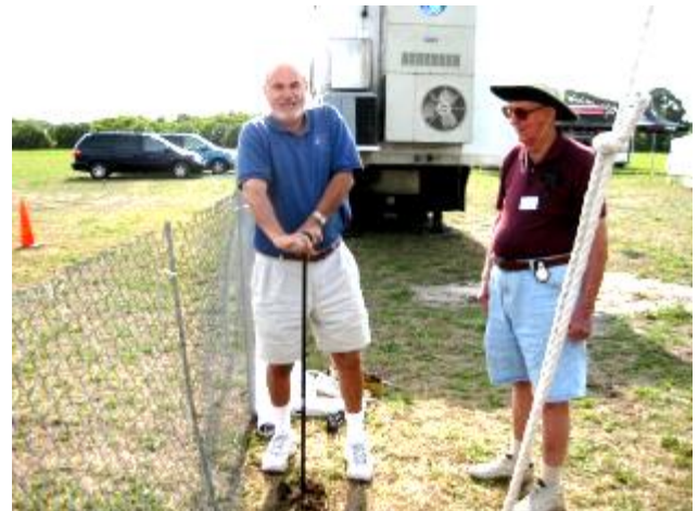
Dil-W8DIL supervises as Bob-K1NOK breaks ground for the antenna mast support.
