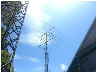
Bob Schneider-W5GJ has an impressive array of antennas at his QTH on the Isle of Venice. On the left can be seen a section of Bob's Hy-Tower vertical used for 80m & 40m; on the right is his 50' US Tower crank-up at about 35' with yagis for 30m through 6m & 2m. Bob also has a wire antenna up for 160m.
