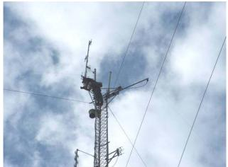
On 24 November, Ron LeBrun-KB4RON repositioned the 2-meter W4AC Repeater antenna to the top of the 200' tower at the Newport Offices site. Previously, the array had been at about 180' AGL. The cantilevered support is for one of the inverted-V HF antennas used by the remote radios at the site.
