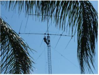
The new beam is in place and Ron begins dressing the antenna's control cable down one tower leg.
