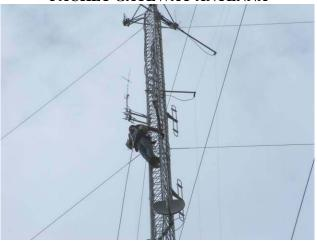
Ron-KB4RON has just installed the 2-meter Ringo Ranger utilized by the packet gateway station at the repeater site.
