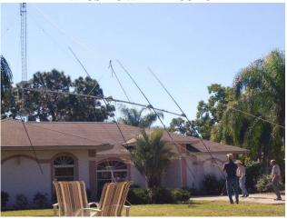
09 November was the BIG DAY, as the 4-element SteppIR beam was ready for installation on the 70' tower. Here, Ron-KB4RON checks the angle and progress of climb, communicating via 2 meters with Julio-W4HY at the electric winch.
