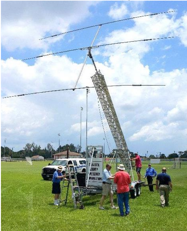
TARC's Jim Shortill-KJ4NDO was there when the mobile Aluma tower with TA-33 tri-band beam was being cranked up to useful status. That's Jim on the left at the head of the trailer.
