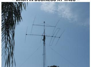
After a void of several months, the beams at W4JS are back in business once again. The 4-element SteppIR was retrofitted with the 30/40 meter driven element which has already proven its worth. Ron LeBrun-KB4RON is up at 70' on the Rohn 45 tower putting the finishing touches on the updated installation. Great job, Ron!!
